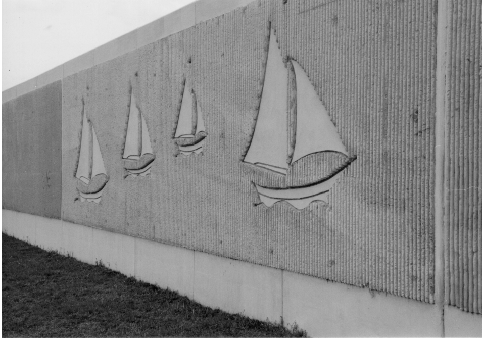
Figure 11-3. Use of fractured ribs highlights artistic design
