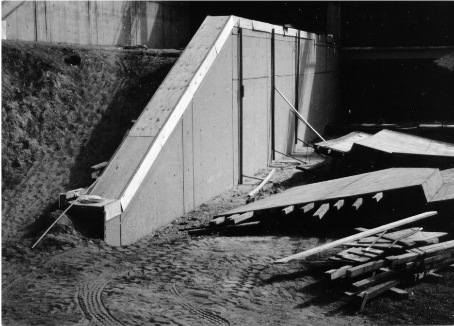
Figure 7-3. Protection of architectural concrete
