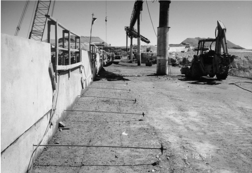
Figure 11-5. Form anchors in RCC placement
