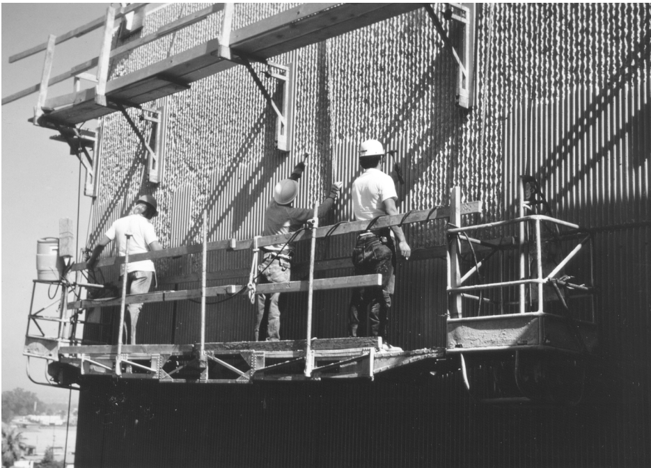
Figure 8-7. Fractured rib texture being developed
