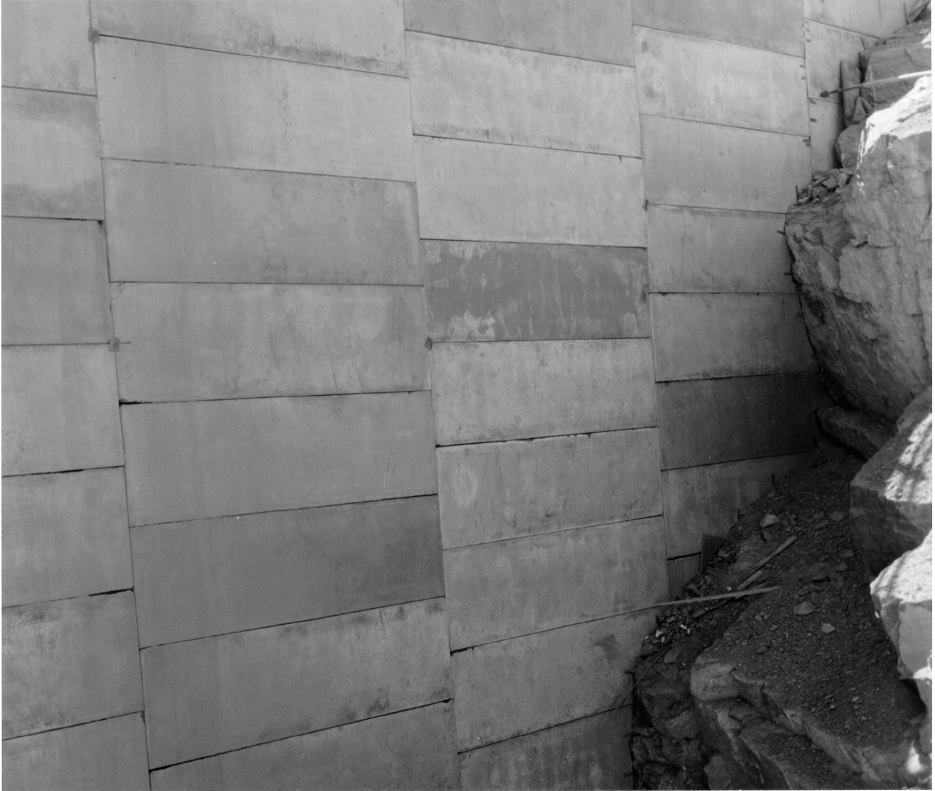
Figure 11-4. Precast concrete forms remain in place in RCC placement
