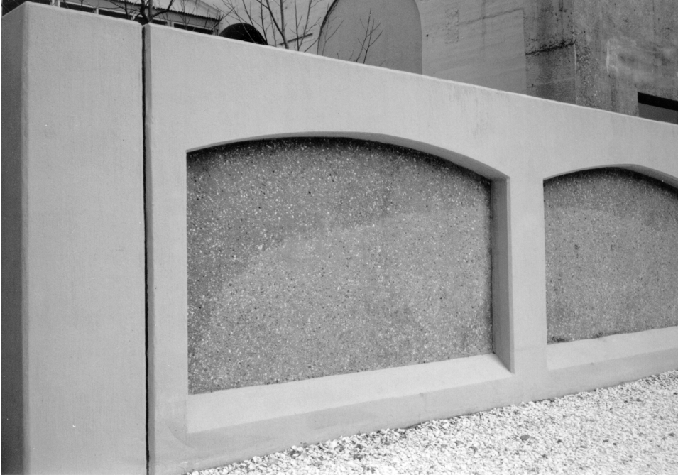
Figure 11-1. Architectural arch design in flood wall
