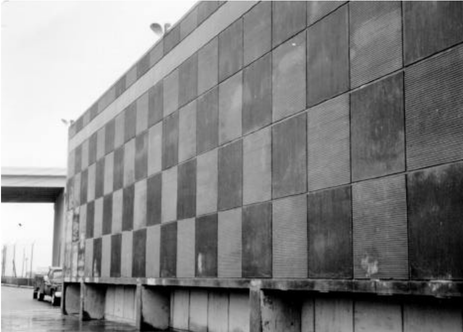
Figure 3-1. Example of an as-cast texture
