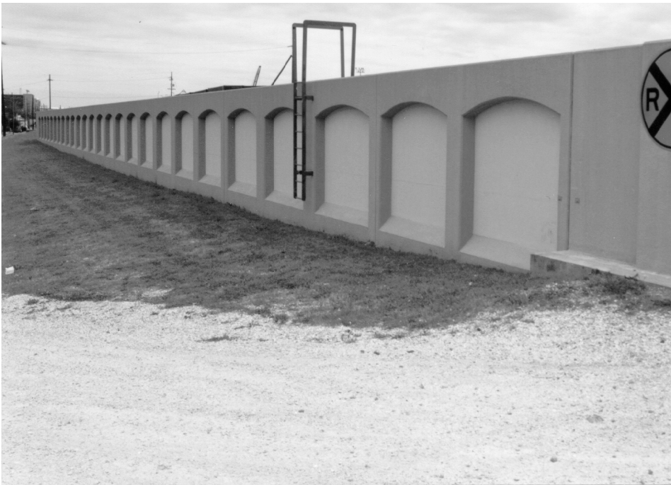
Figure 11-2. Painting of concrete highlights arches in floodwall
